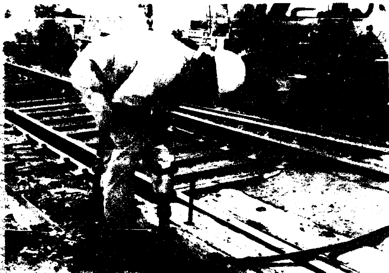
FRANK SLABY PREPARES CONRAIL CROSSINGS for revamping in the stretch between Dexter and Chelsea. He uses an impact wrench to unscrew guard legs (and later secure them again) at the crossings. Conrail's construction project scheduled for the summer of '86 will replace the main rail on the south side with new welded rail designed to permit faster travel by Conrail trains. Several Conrail crews will continue to work in the Chelsea and Dexter areas until September.
